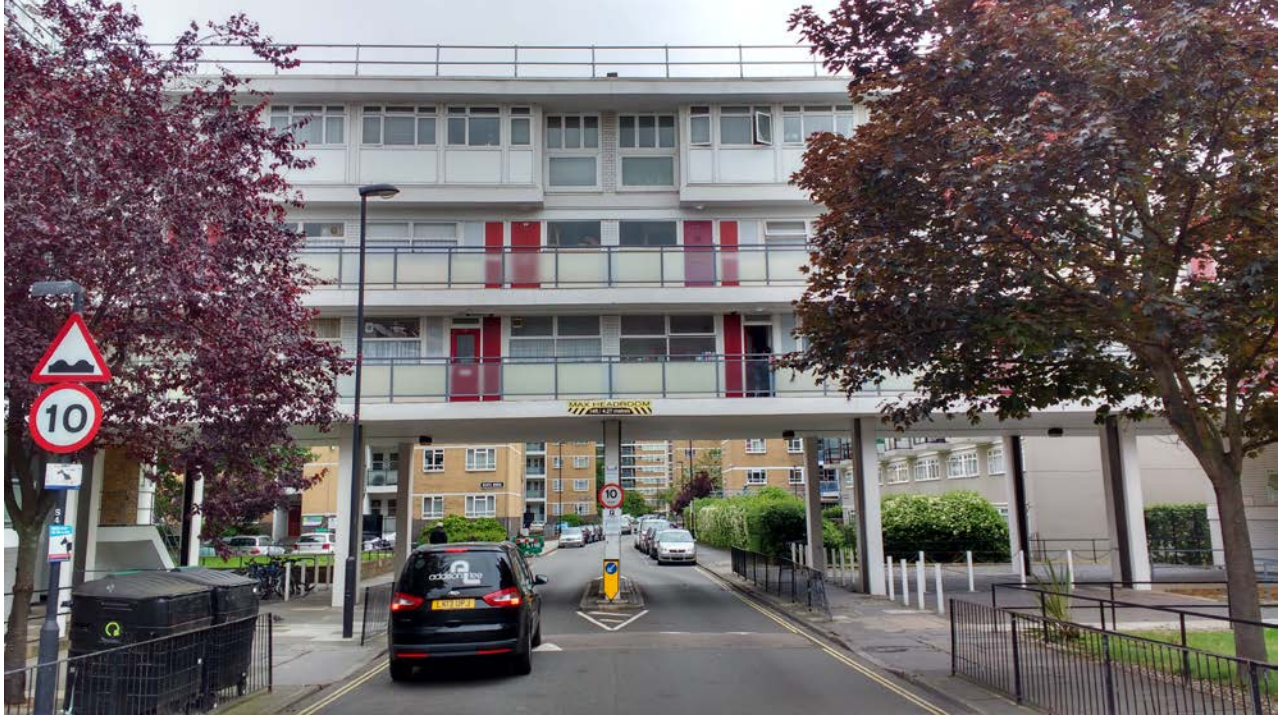
View of Moyle House from Churchill Gardens Road
